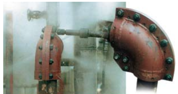
Leak Seal Box Fitted and Sealant Being Injected
